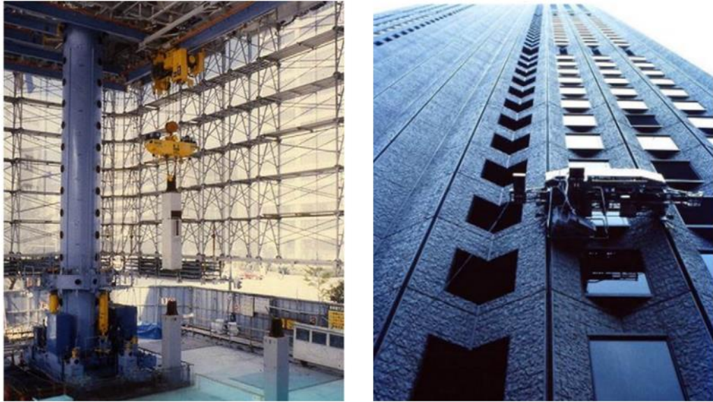
Figure 2.5 Left: Robot-oriented design in an automated construction site. Right: Single-task construction robot painting a façade. (Bock, 2015)
