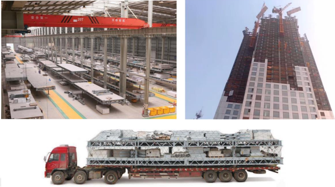
Figure 2.7 Top left: Prefabrication assembly line. Top right: Assembly of Mini Sky Tower. Bottom: Transportation of prefabricated components. (Generalova et al., 2016)
