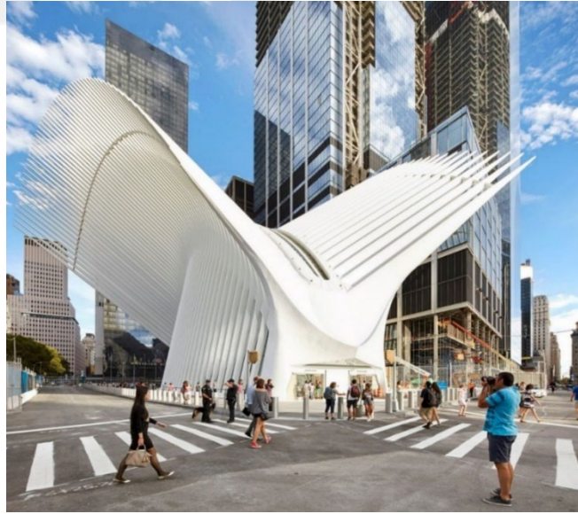
Şekil 3.24 : World Trade Center Transportation Hub, Santiago Calatrava, 2003-2016, ABD (Hufton & Crow, 2017).
